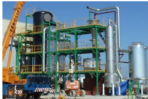
Woodchips Gasification Co-Generation. 2.0 Mwe. Ejea de los Caballeros, Spain
