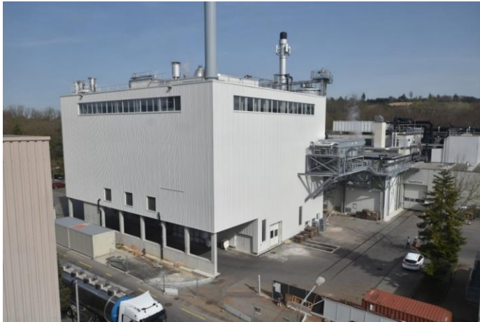
MBM Gasification 18 MWth. Lyss, Switzerland
